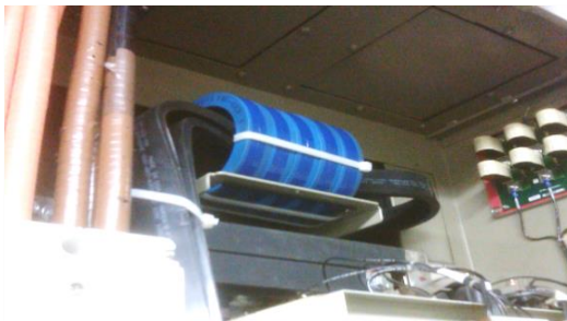
Installation Example #3 – Flat Wire
