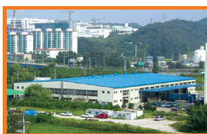
Head Office and Factory - 1
