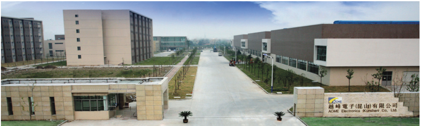
ACME Electronics (Kunshan) Co., Ltd., Jiang-Su Province, China
